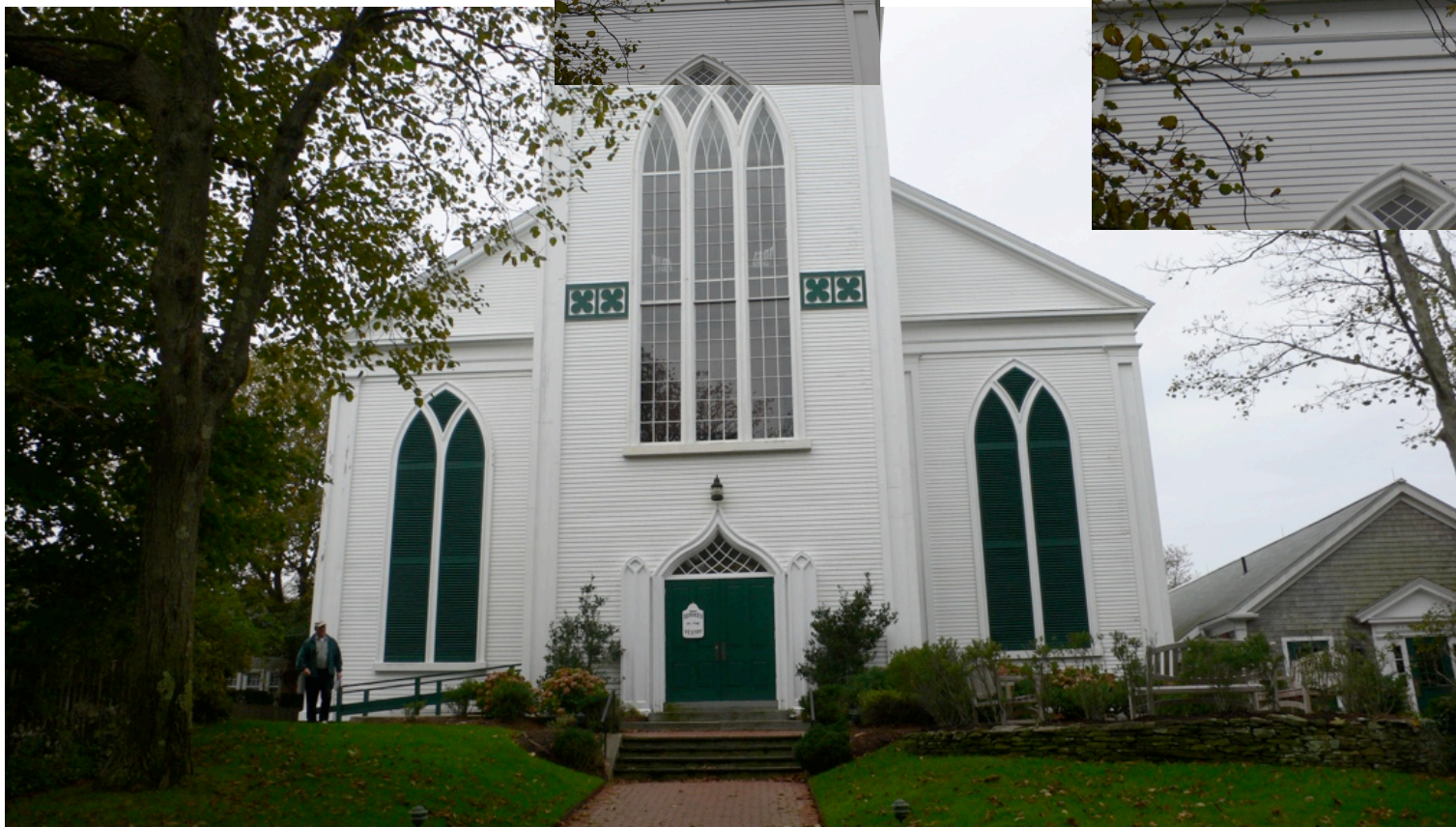
East facade of church, composite view
