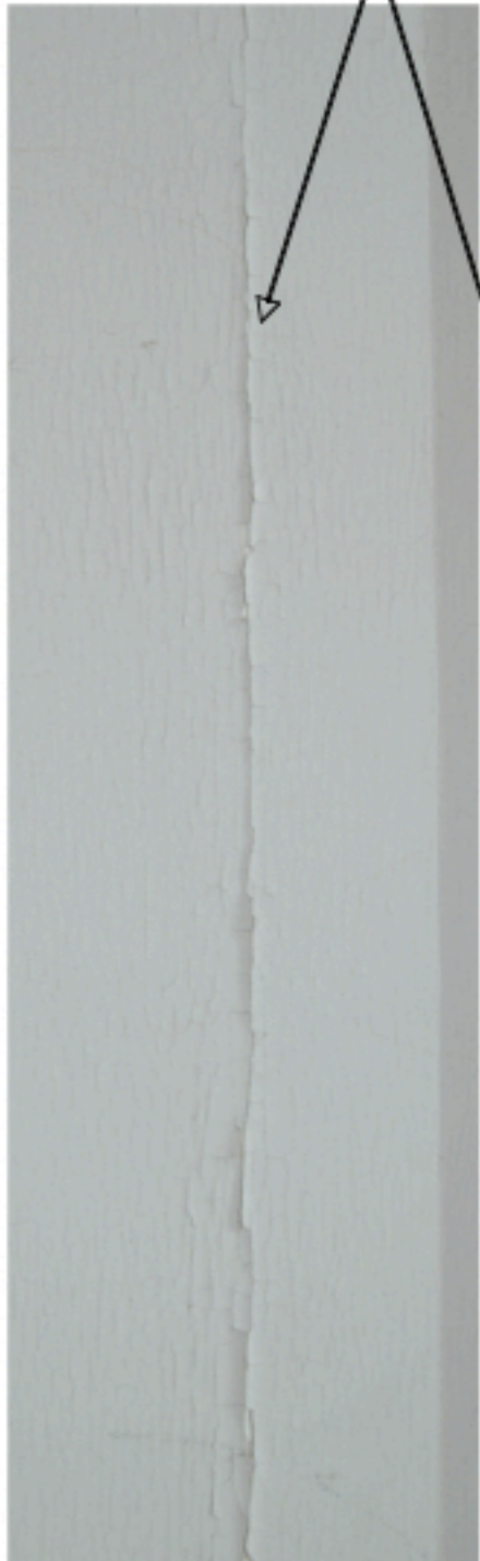
Interior Cracks and Peeling
