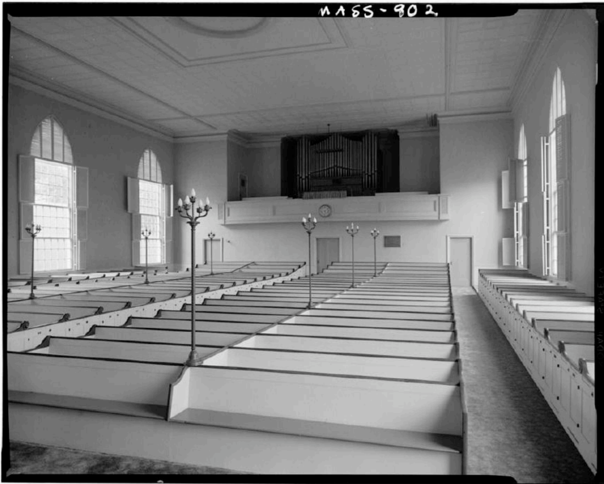
7. Historic American Buildings Survey Cortlandt V. D. Hubbard, Photographer July 1966 INTERIOR, EAST END, BEFORE RESTORATION HABS MASS,10-NANT,26-7
