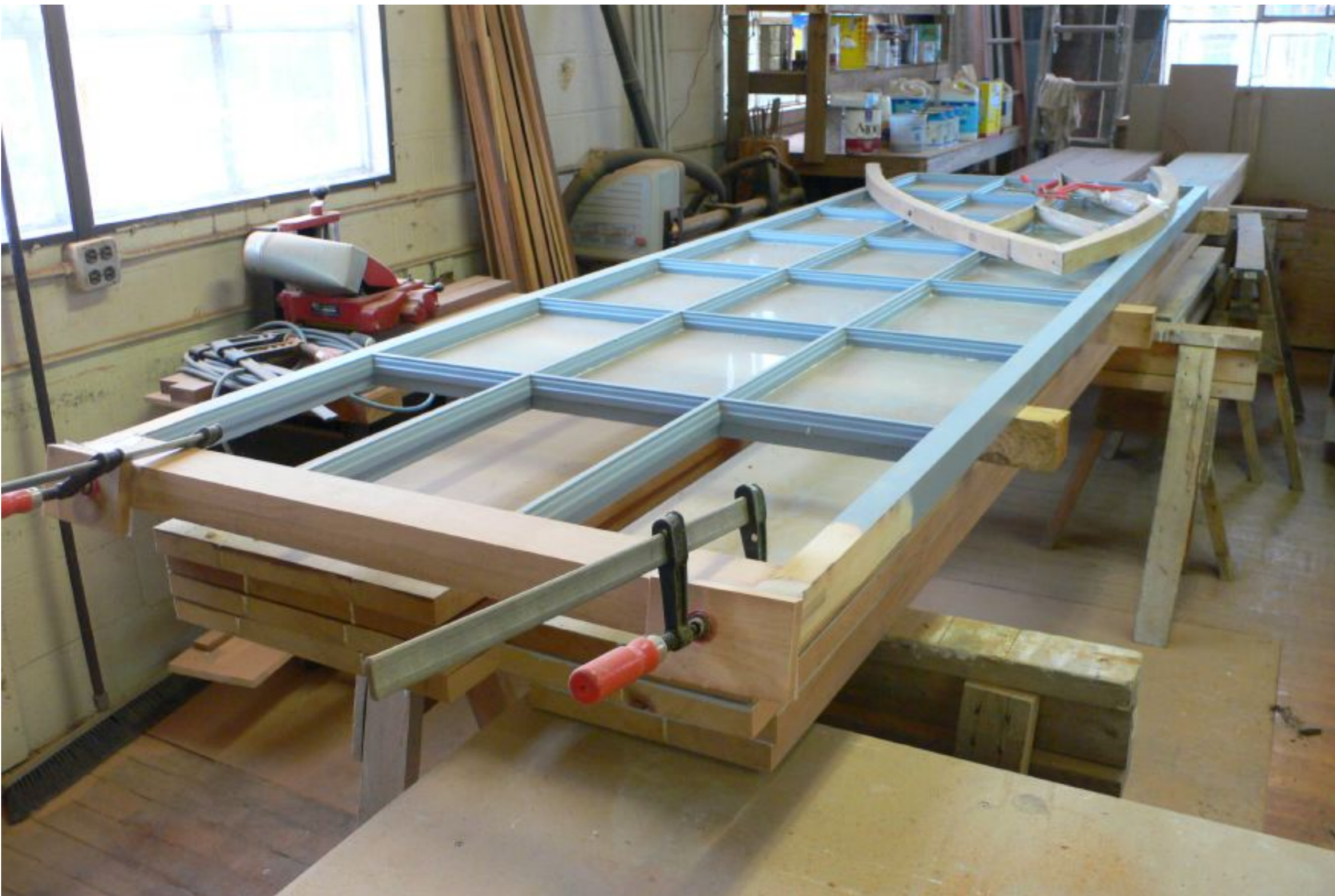
Rectangular window, repairs to deterioration at bottom rail in process
