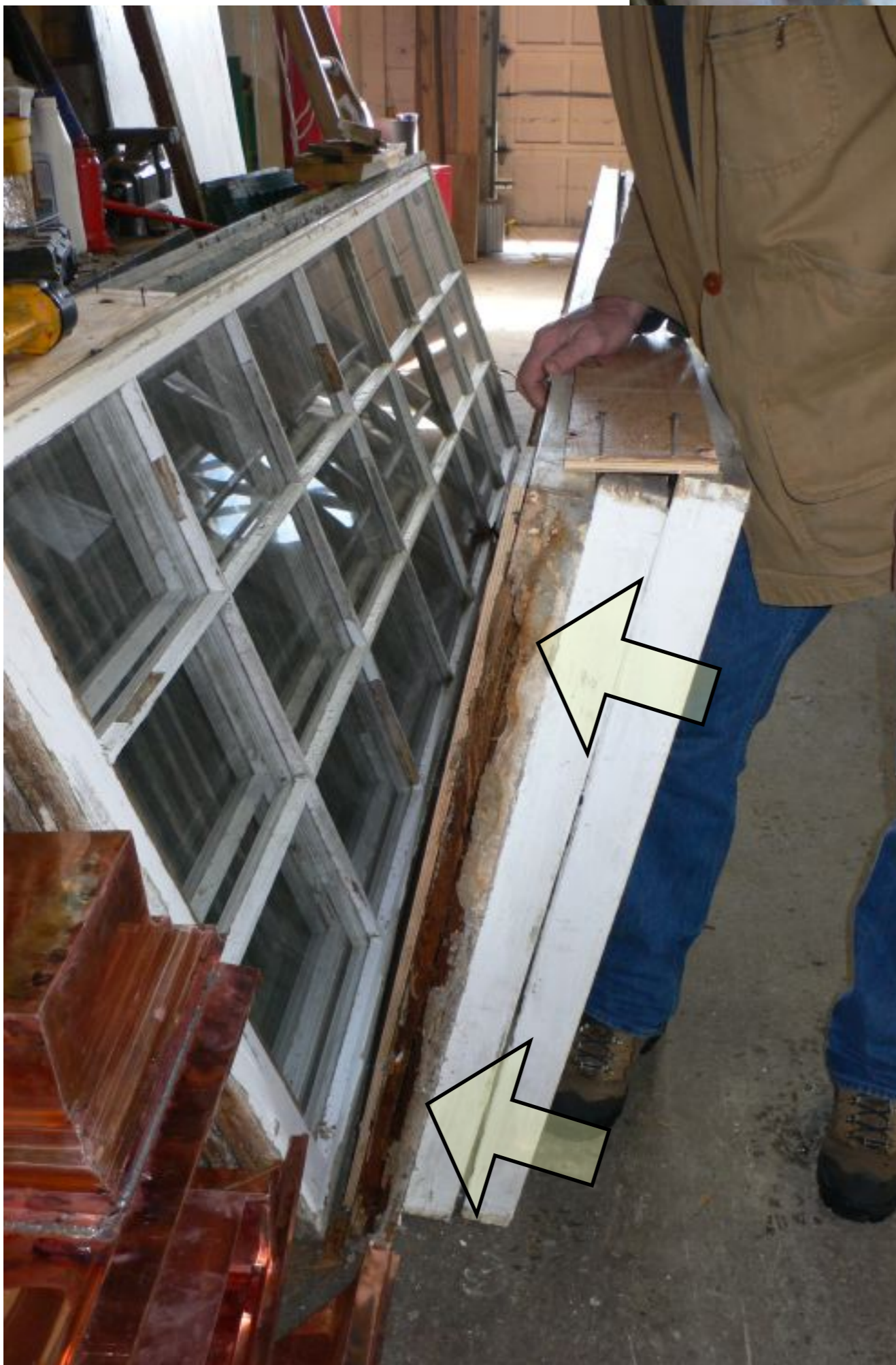
Rectangular window deterioration at bottom rail
