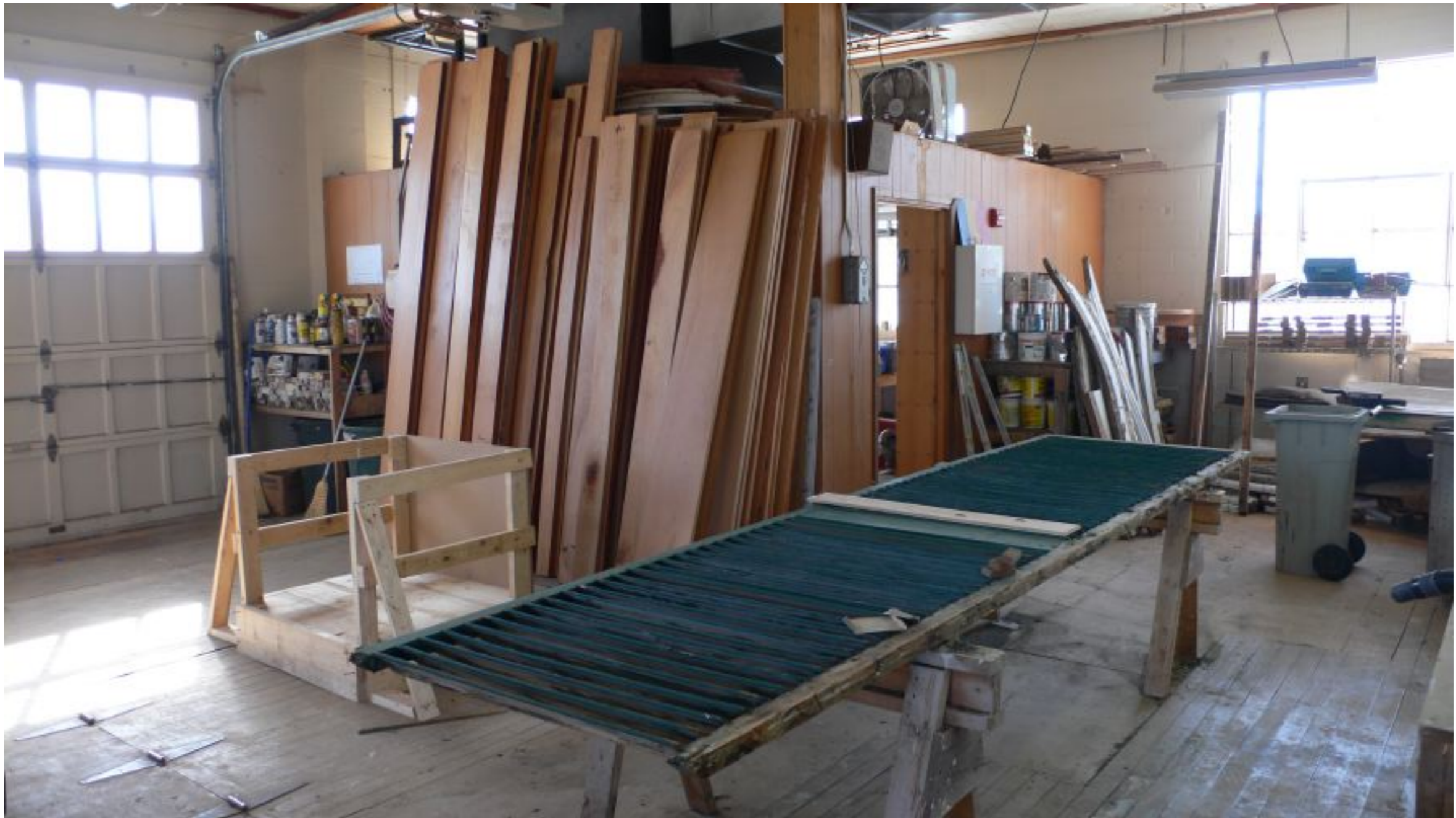
Louver conservation underway with stockpiled mahogany in background
